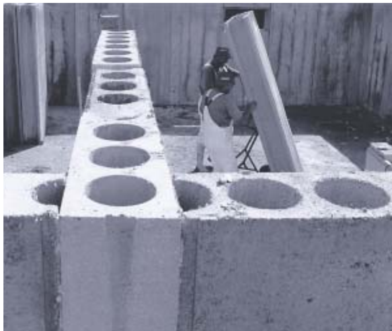
Lichtbeton van EPS (foto BASF).
